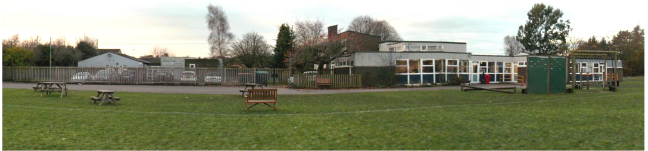
Existing north elevation of the school
